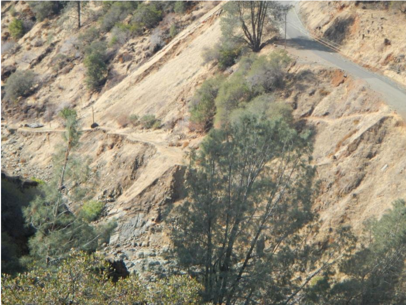
Figure 4: Photo of Narrows 2 access road and erosion scars (Oct. 30, 2014).
