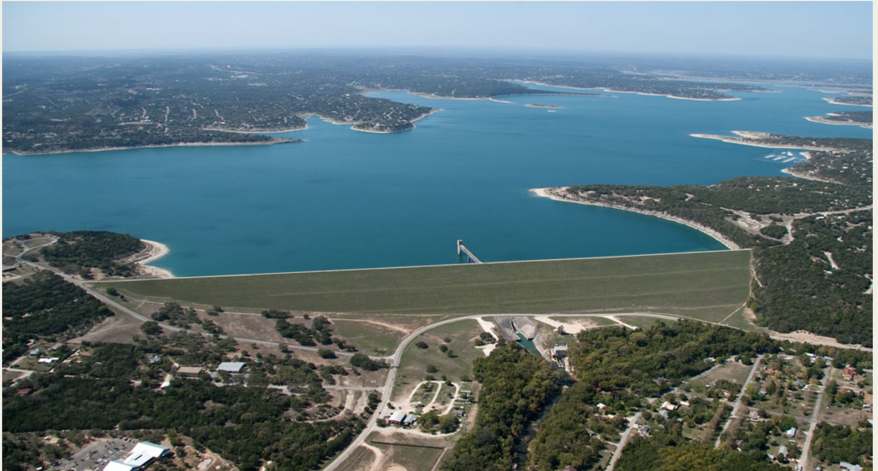
Canyon Lake Dam and the Guadalupe River, TX - photo from edwardsaquifer.net
