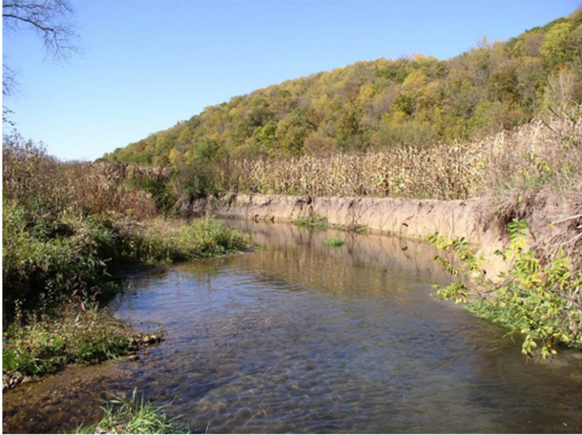
Streambank erosion prior to restoration on Big Spring Branch, Wisconsin. Photo by Nohr Chapter of Trout Unlimited.
