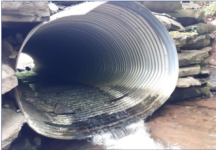
Batavia Kill - Barrier #4 at Sherwood Road
