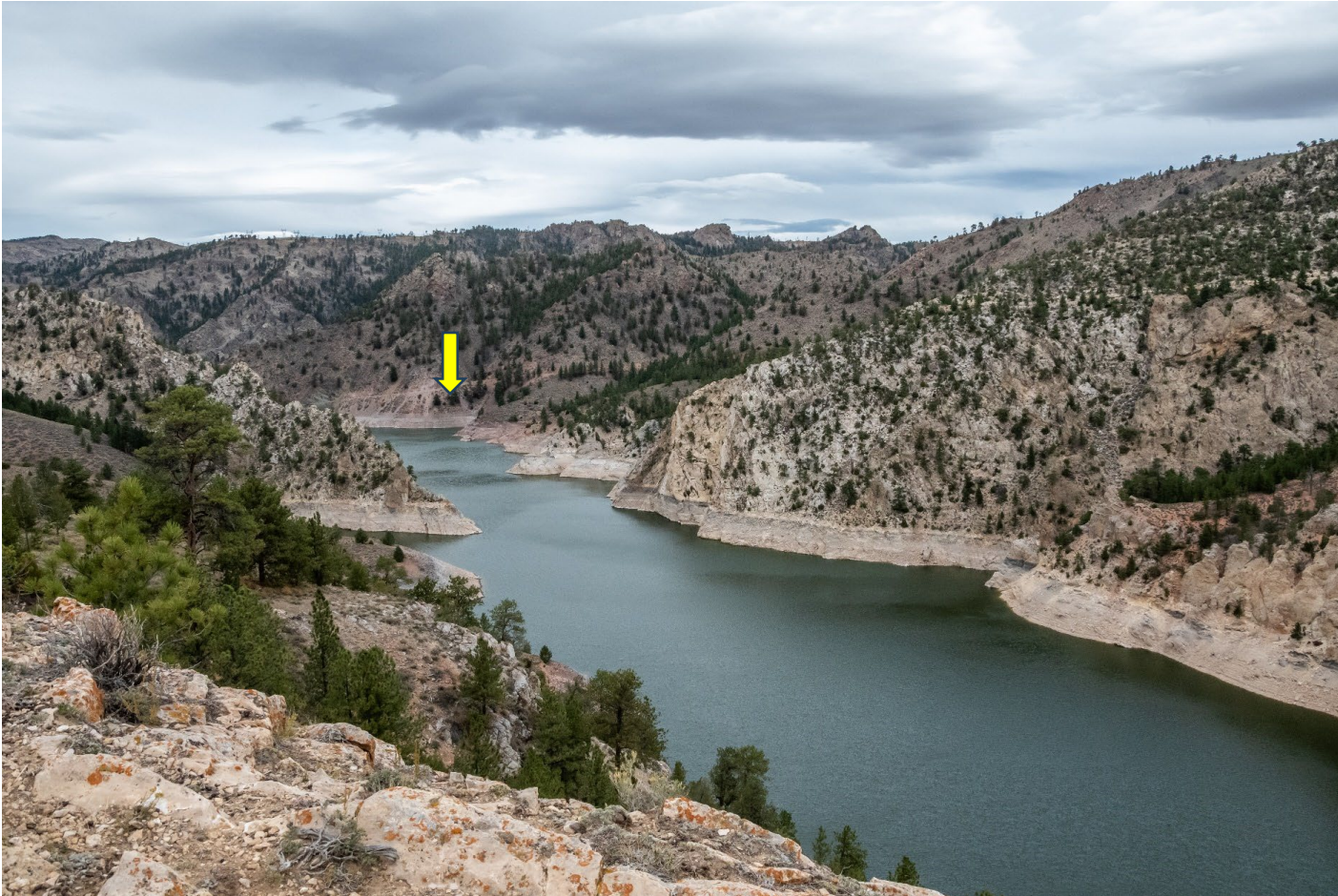
Figure 5. View of Seminoe Reservoir looking towards location of proposed lower intake structure (source: Appendix K of BCH's license application).
