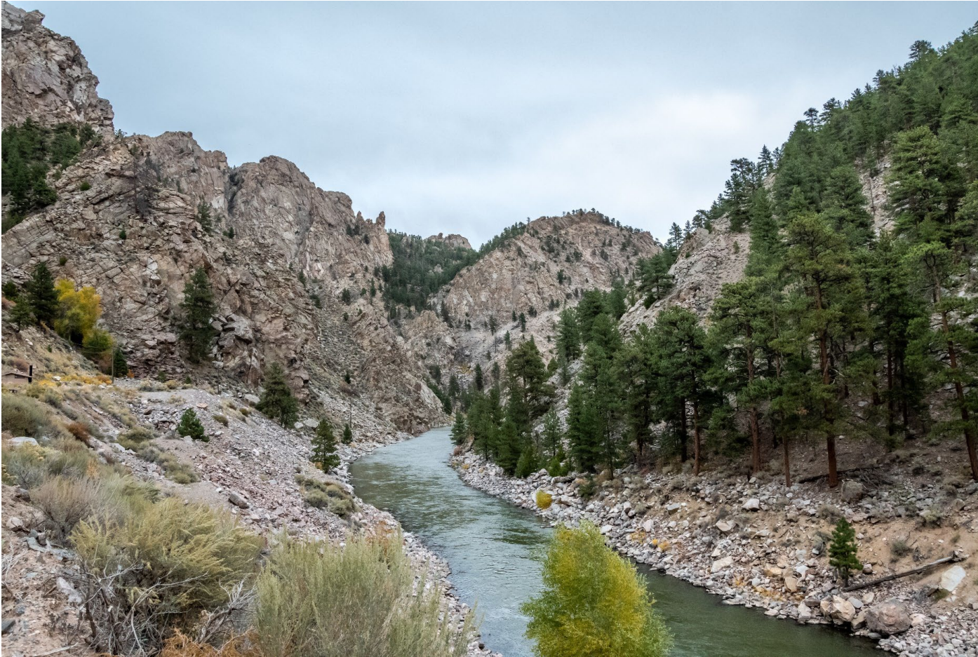
Figure 7. View of Seminole Dam tailrace looking towards location of the proposed bridge connecting to the main access tunnel (source: Appendix K of BCH's license application).
